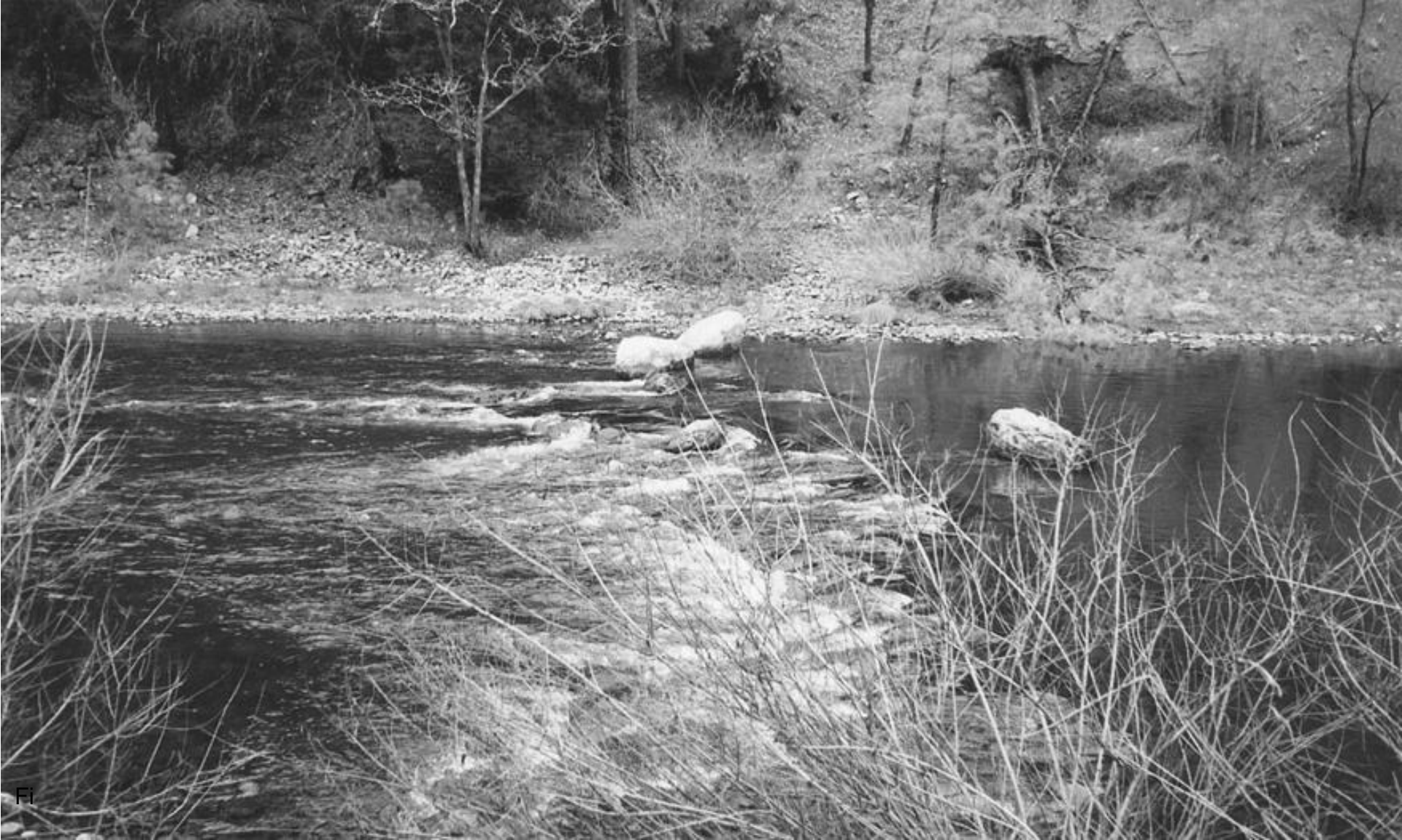
Artificial riffles designed to create spawning habitat by creating the forms, Trinity River
