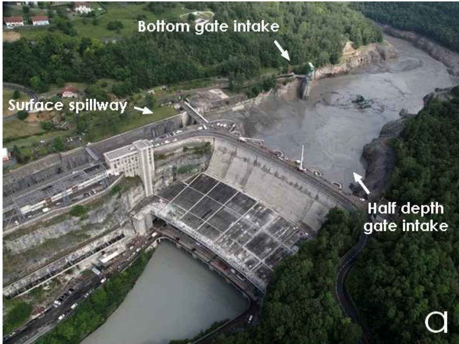
Génissiat dam during the 2012 flushing operation
